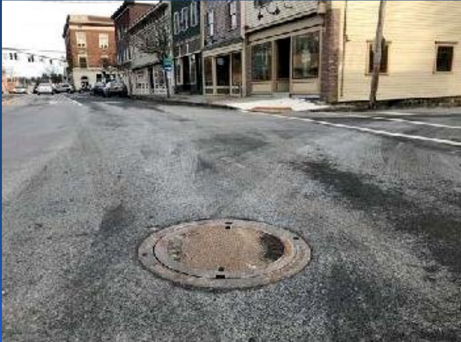
Self-Level Manhole After 2 Years
