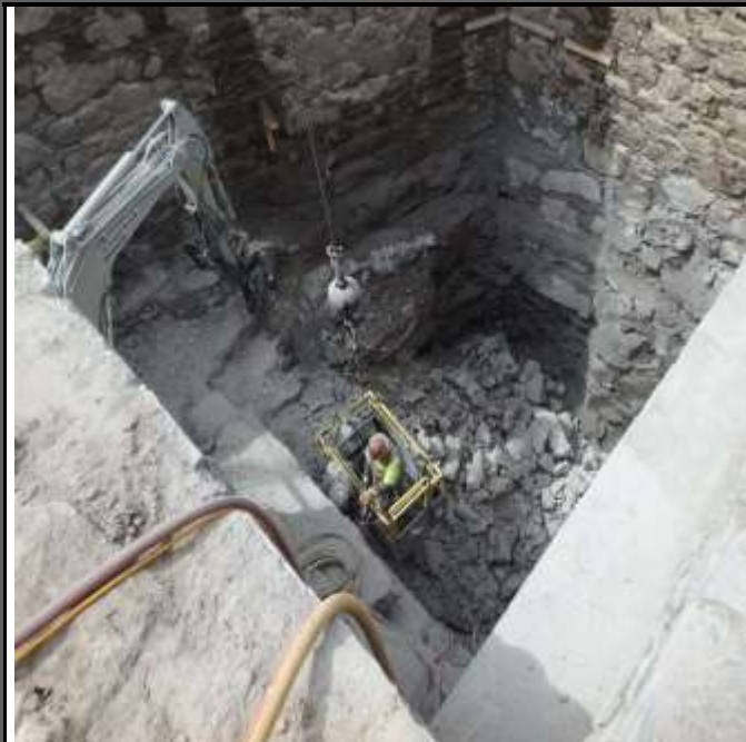
View of the pit as the crew Drills, Splits, and chips. (5-11-17)
