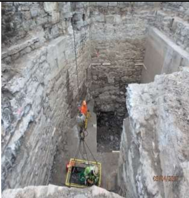
View of the pit from above the penstock tunnel as the crew is surveying and excavating (5-04-17).
