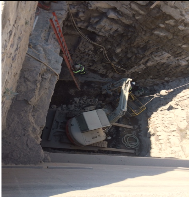
Looking into the pit from the north wall as the excavator is used to help with the chipping process (7-30-17).
