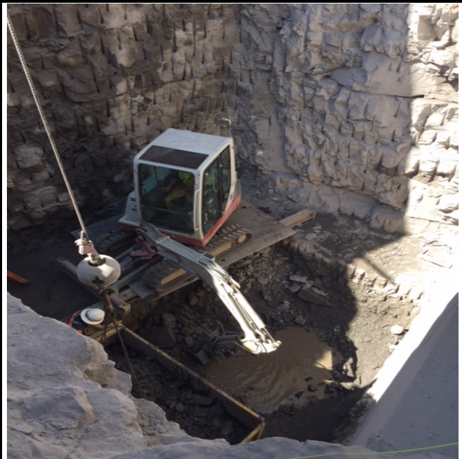
View into the pit from the north wall. The crew is mucking out the lower pit (7-31-17).
