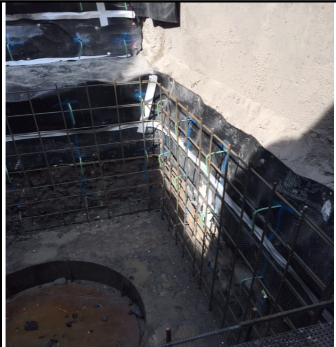
Rebar has been installed in the lower pit (8-10-17).
