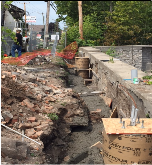
Concrete has been placed in both the trench and the Sonotubes (8-11-17).
