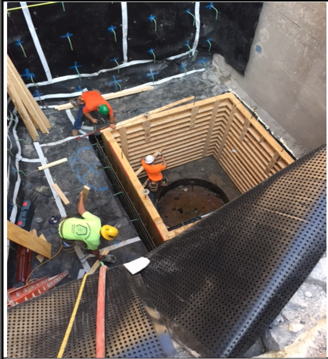
The Carpenters are working on installing the formwork in the lower pit (8-12-17).
