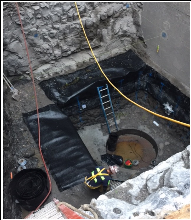
The crew has begun installing water board (8-08-17).
