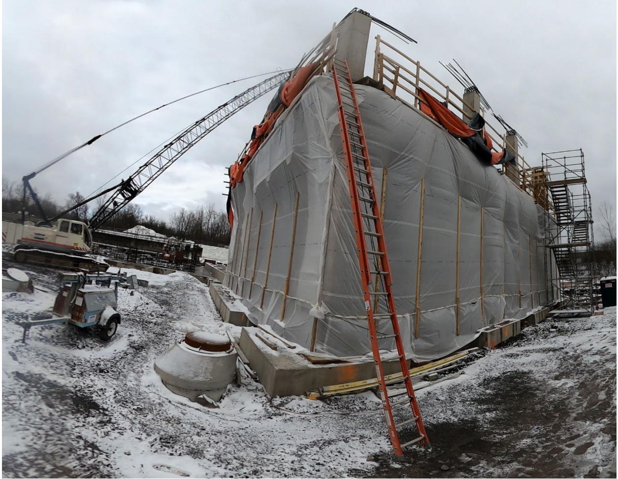
Dewatering and Dryer Building (2 nd Story Floor Slab Cold Weather Concrete Protection)
