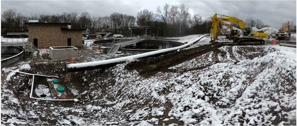
Bypass Piping Staging
