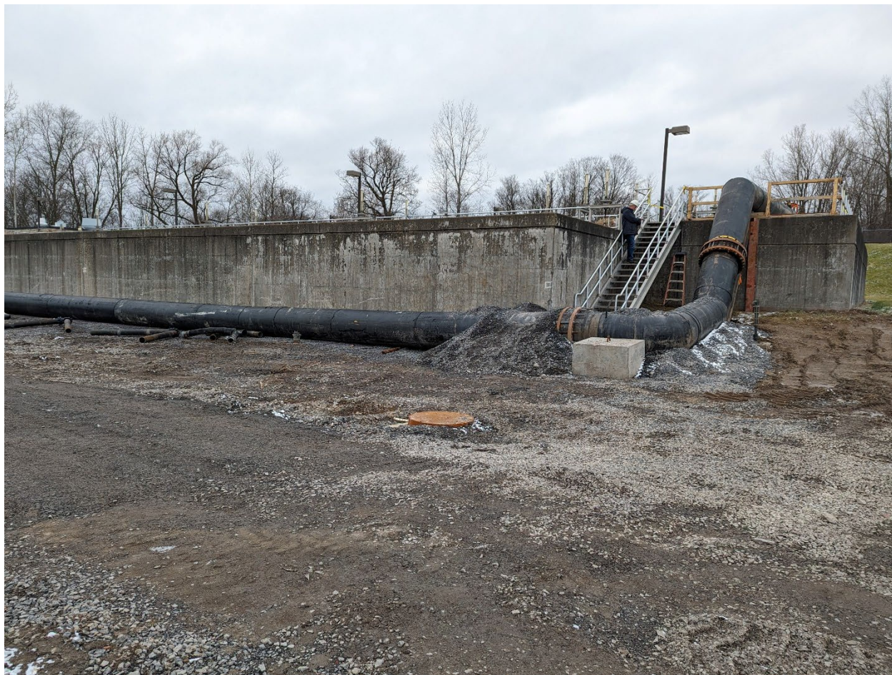
ABOVE: Primary Effluent Bypass Piping Discharge into Aeration Tank (Secondary Treatment)
