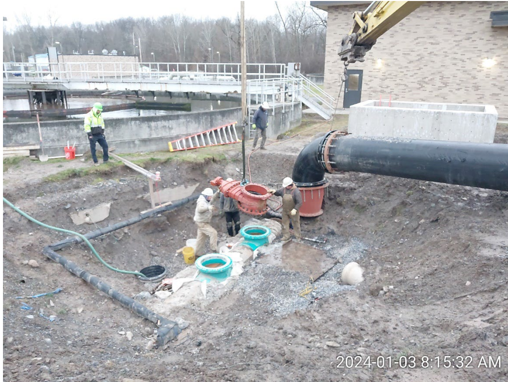
ABOVE: Primary Effluent Bypass Piping Preparations
