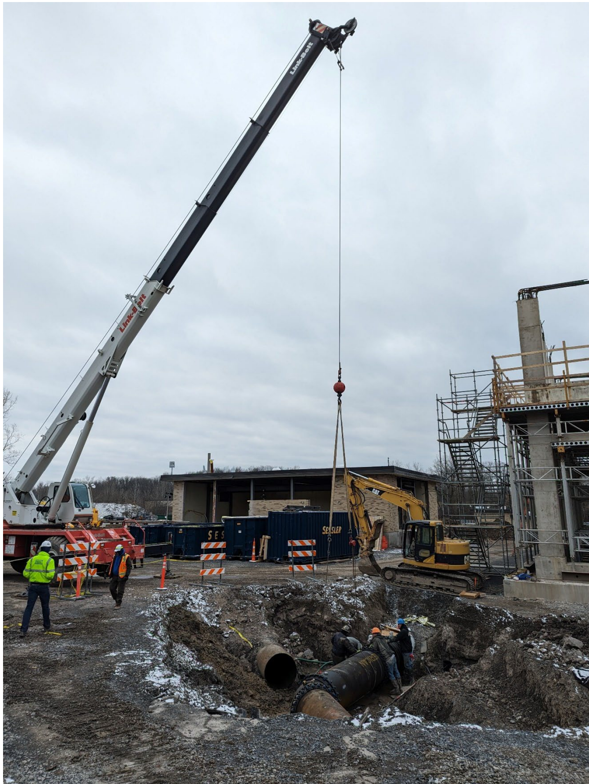
ABOVE: New 36" Primary Effluent pipeline is reconnected to the existing pipeline, completing the redirection of flow; concrete thrust block added behind pipe elbow after bolts tightened
