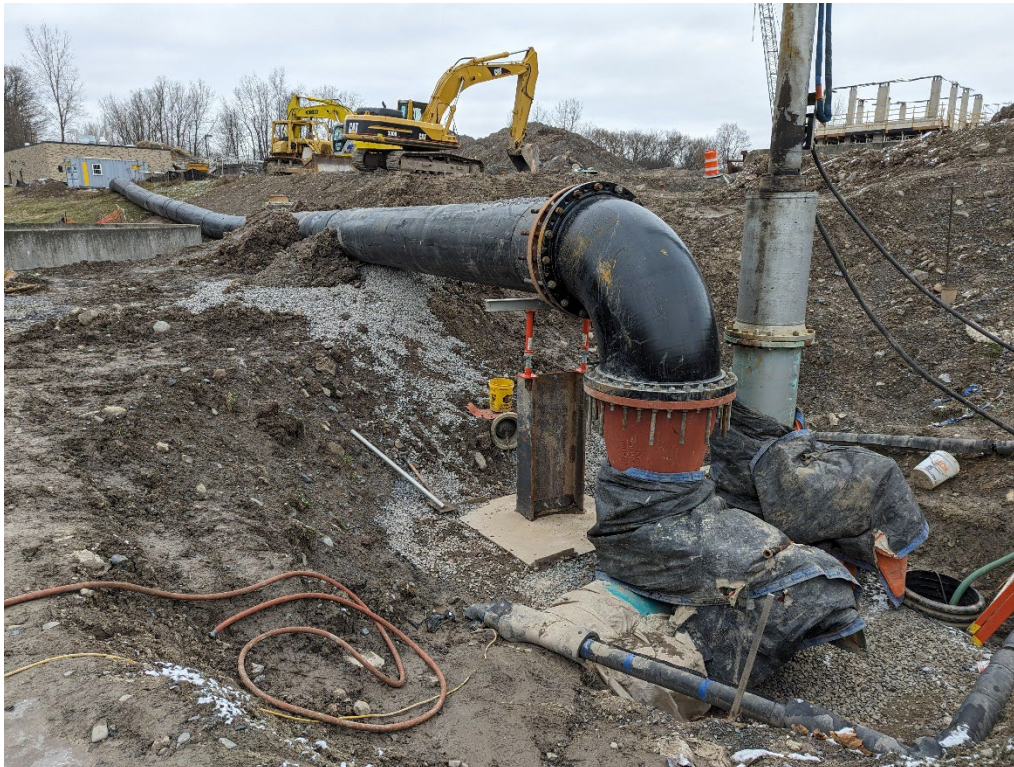
BELOW: Bypass Installed; Line Stop (gray cylinder) is next to piping and shuts down flow within the pipe creating the flow diversion through the bypass
