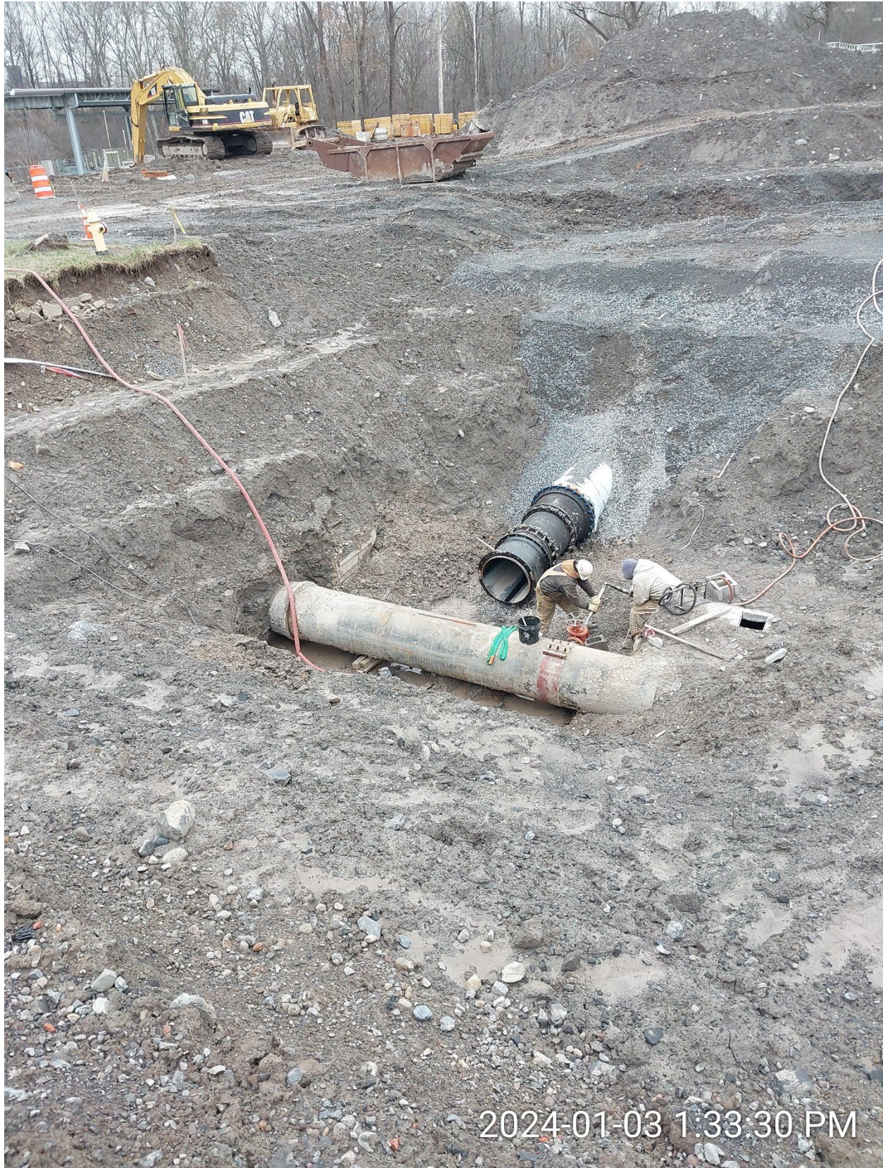
ABOVE: New Primary Effluent Pipeline ready to be connected to existing once bypass is active BELOW: Connection completed; the pipe then receives a concrete thrust block in the void behind the elbow for restraint and then backfilled
