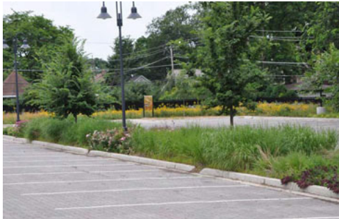
This parking lot has permeable paving and a bioswale which significantly reduce the runoff that is directed towards the stormwater system.
