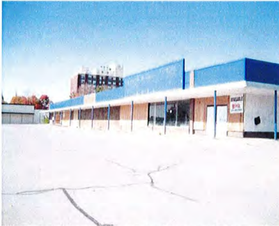
View of subject property, looking west from Nelson Street.
