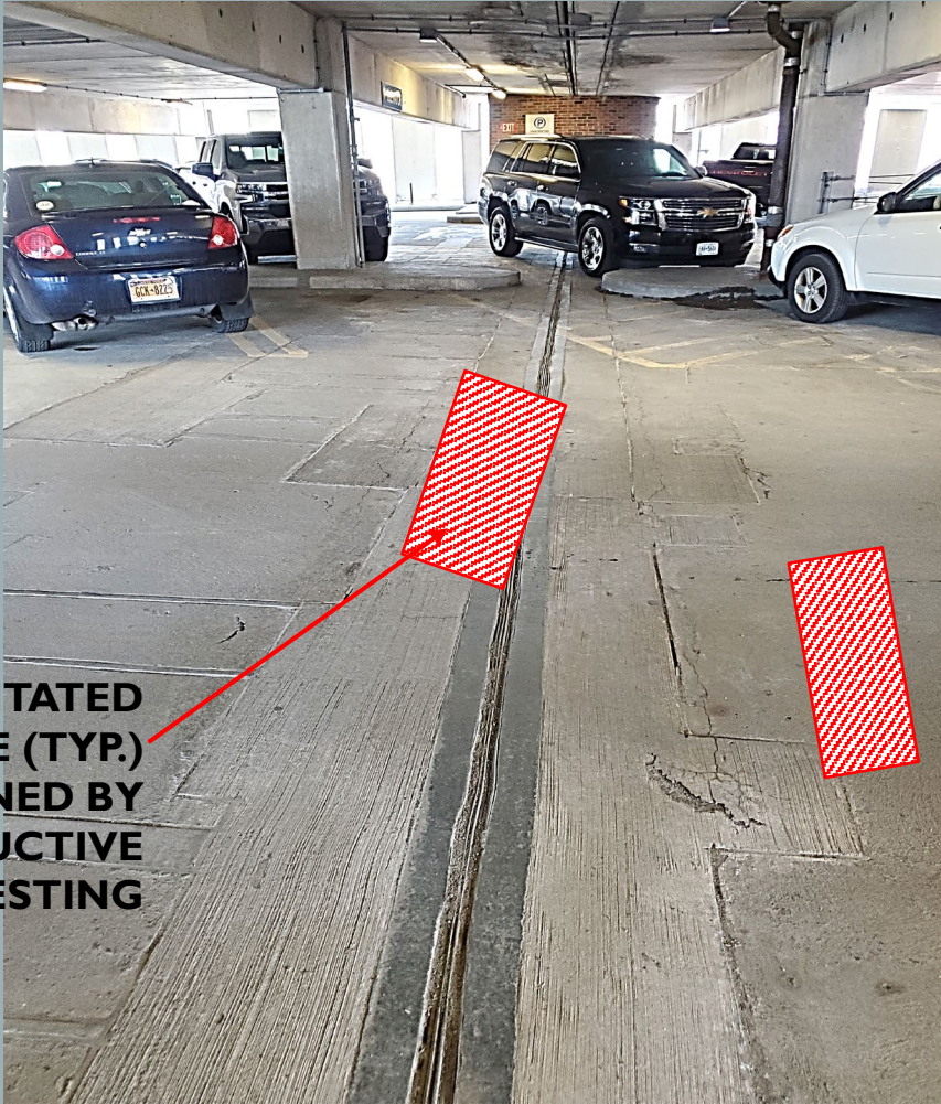
DELAMINATED CONCRETE NOTED DURING INSPECTION AT EXPANSION JOINTS
