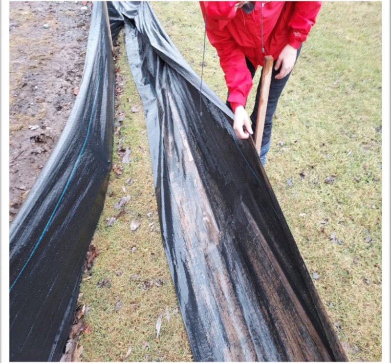
Monitoring the installation of erosion control products and addressing failures.
