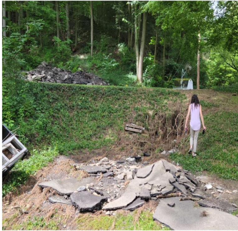
Responding to severe erosion following a storm event in August of 2021.
