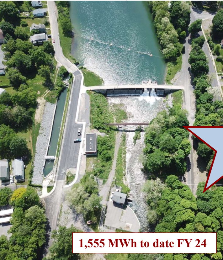
Mill Street Hydro
