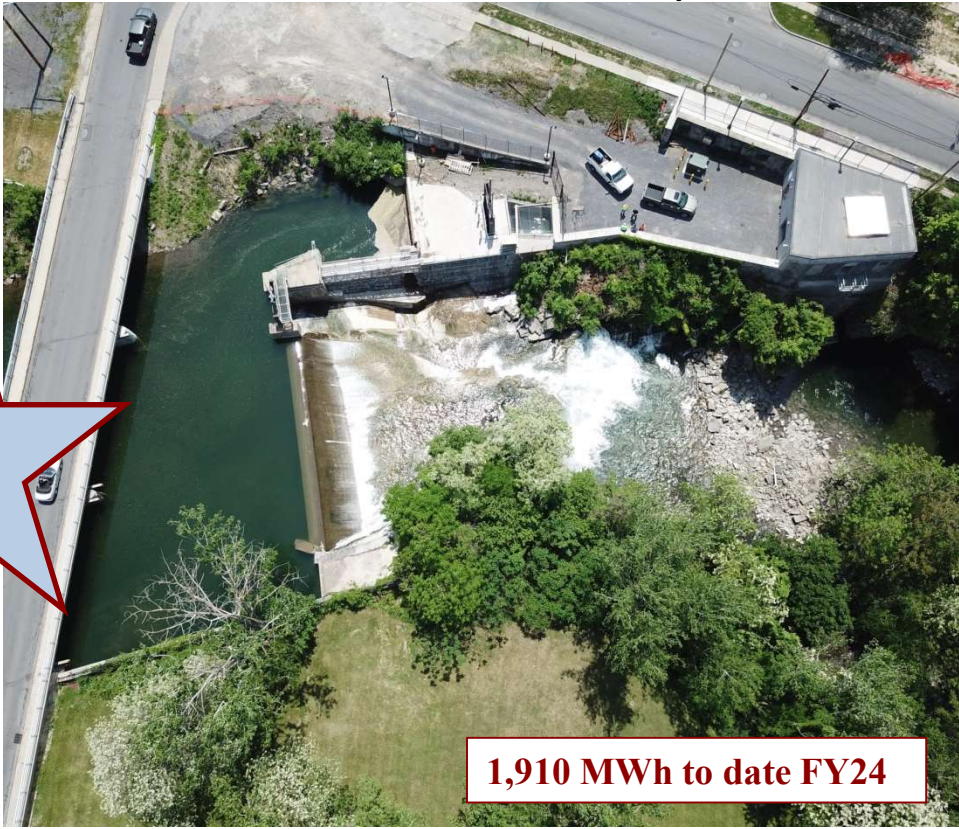
North Division Street Hydro
